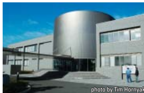
photo by Tim Hornyak Kochi Core Center's main building
