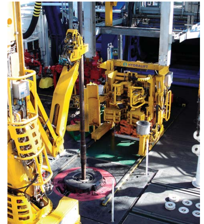
Central area of the drill floor. The assembled drill pipe was passed down through the floor, and joined with the power slip on the floor surface.
