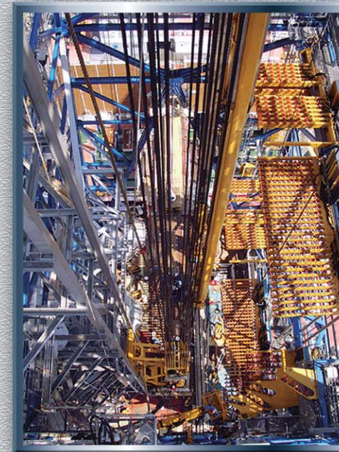
By winding the wire cable back and forth over eight pulleys between the Derrick Top and the Top Drive, the load applied to the cable is reduced by one-sixteenth of the actual load.
