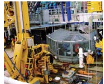
The rig floor with the drilling equipment is lined up and ready for operations is a symbol of the group's collaborative effort.
