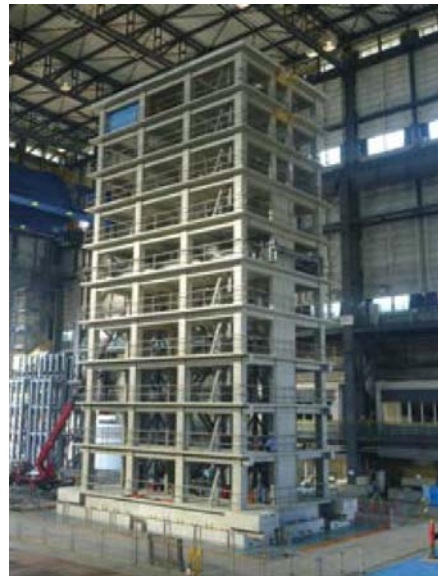
Fig. 3 Full-scale, height 27.45m 10-story RC building.
